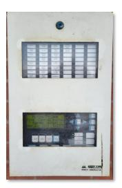
The building is equipped with a **Mircom** system. In case of primary power failure, the system automatically switches to back up power supplied by the battery pack located in the Fire Alarm Panel.
